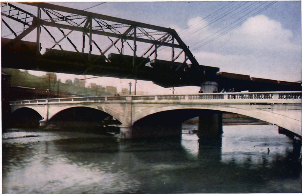
SOUTH THIRD STREET BRIDGE OVER LEHIGH RIVER, EASTON, PENNSYLVANIA Three spans of 92 to 105 feet. Roadway 62 feet. Footings on rock. For the Board of Commissioners of Northampton County, Easton, Pennsylvania, 1912. Illustrating three intersecting lines of transportation.
