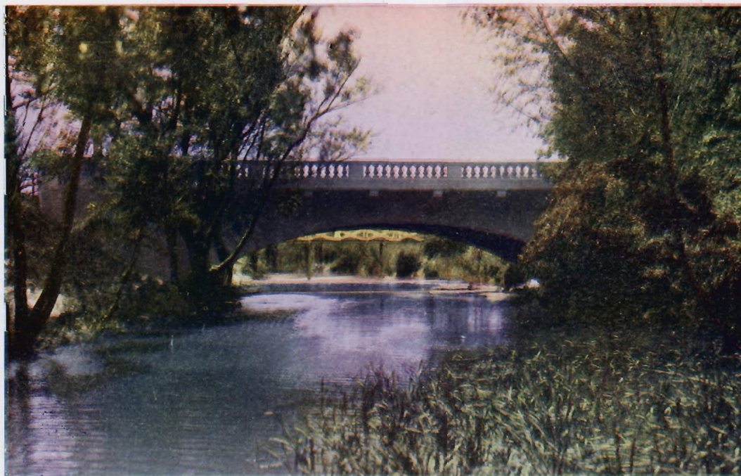
MOCKING BIRD LANE BRIDGE, OVER TURTLE CREEK, HIGHLAND PARK, TEXAS Span of waterway 55 feet. Roadway 30 feet. Footings on rock. For the Town of Highland Park, Texas, 1923.
