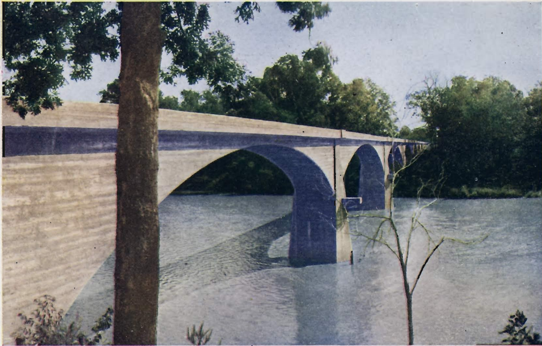
SPRING RIVER BRIDGE, WEBB CITY, MISSOURI Twenty-two spans of 50 to 75 feet. Roadway 11 feet. Footings on piling in clay. For the Southwest Missouri Railroad Company, Baxter Springs, Kansas, 1917. Entire structure completed in three months.
