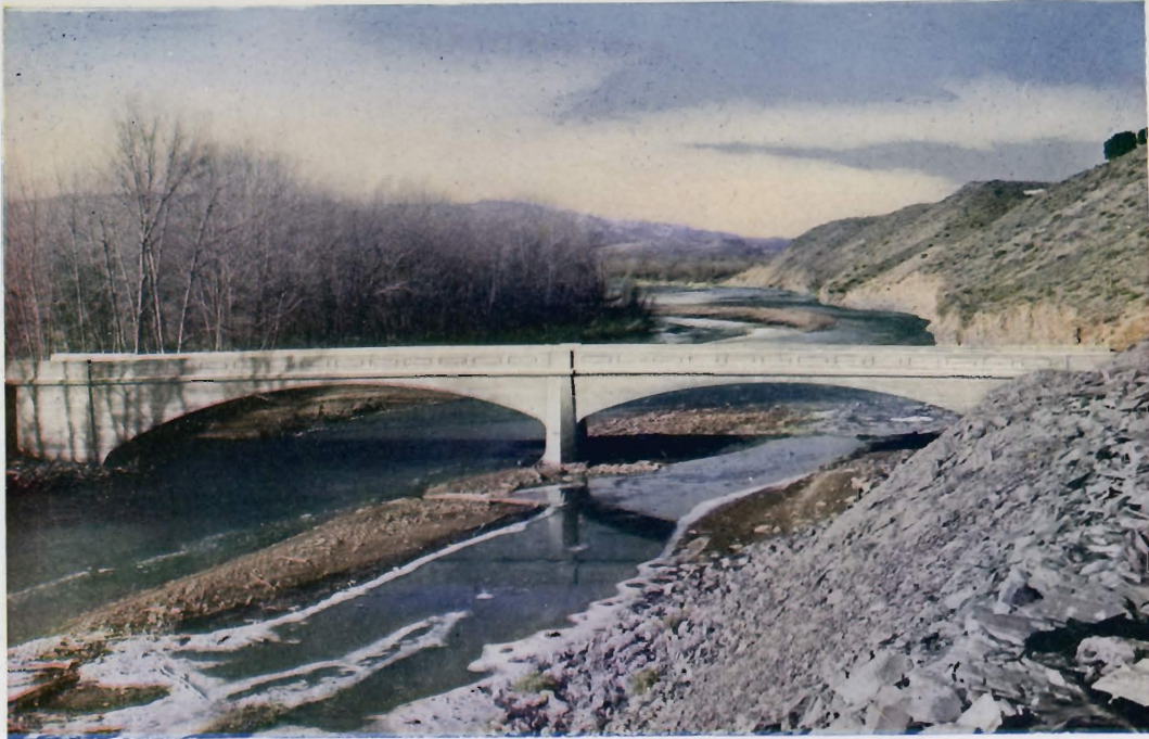
FLORENCE BRIDGE OVER ARKANSAS RIVER, FLORENCE, COLORADO Twin spans of 65 feet each. Roadway 16 feet. Footings on gravel. For the Board of Commissioners of Fremont County, Canon City, Colorado, 1913.
