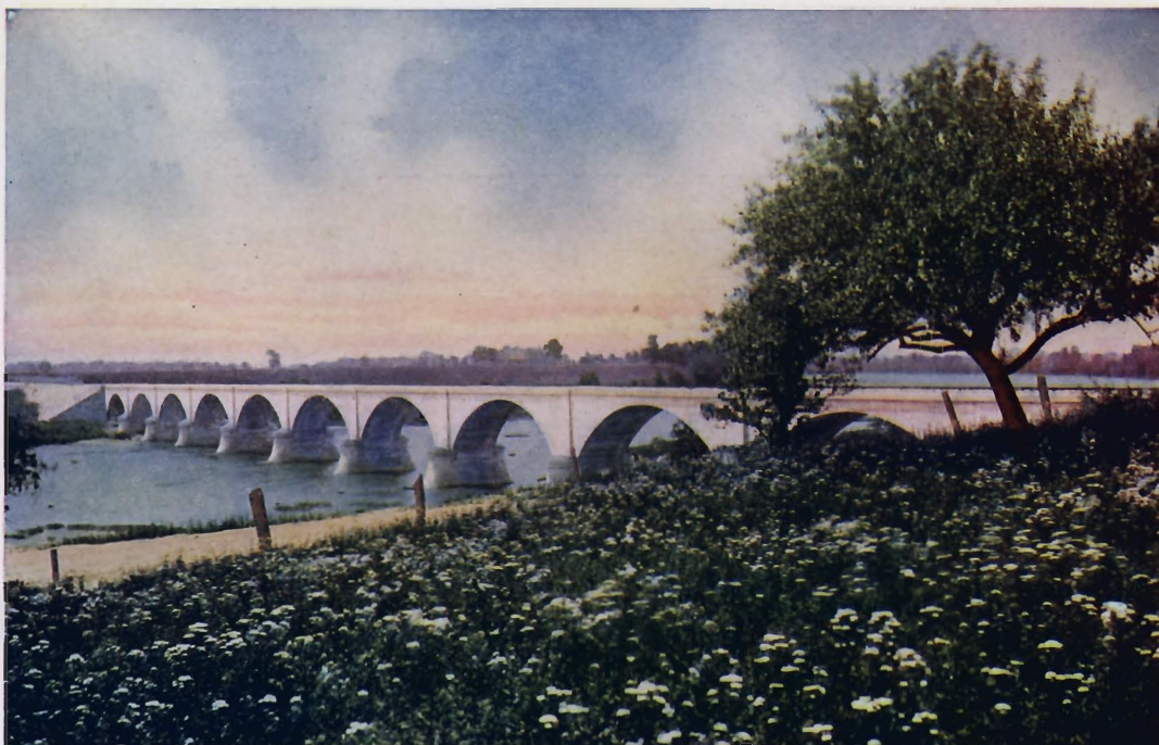
MAUMEE RIVER BRIDGE, WATERVILLE, OHIO Twelve spans of 75 to 90 feet. Roadway 16 feet. Footings on rock. For the Ohio Electric Railway Company, Cincinnati, Ohio, 1907. Other views below and on page 7.
