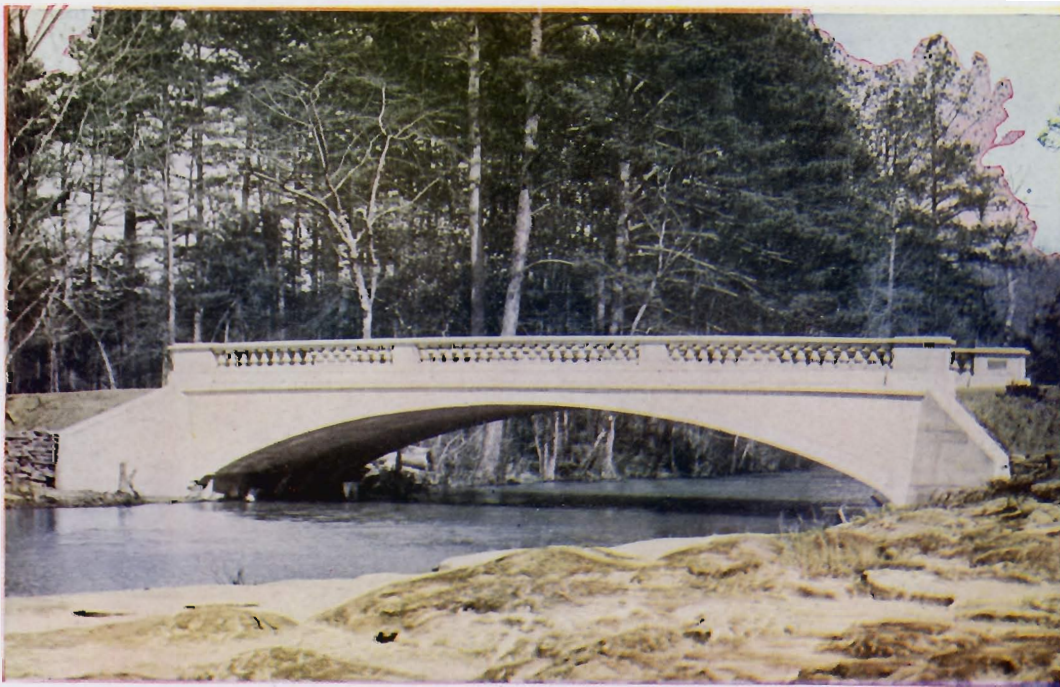
NOCCALULA FALLS BRIDGE OVER BLACK CREEK, GADSDEN, ALABAMA Span of waterway 56 feet. Roadway 18 feet. Footings on rock. For the County Court of Etowah County, Gadsden, Alabama, 1916.
