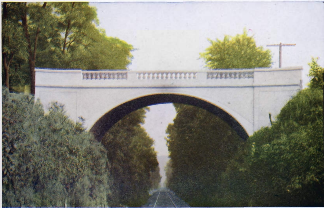
MADISON HILL BRIDGE OVER PENNSYLVANIA RAILROAD, MADISON, INDIANA Span of opening 36 feet. Roadway 16 feet. Footings on rock. For the Board of Trustees of the Southeastern Hospital for the Insane, Madison, Indiana, 1921.
