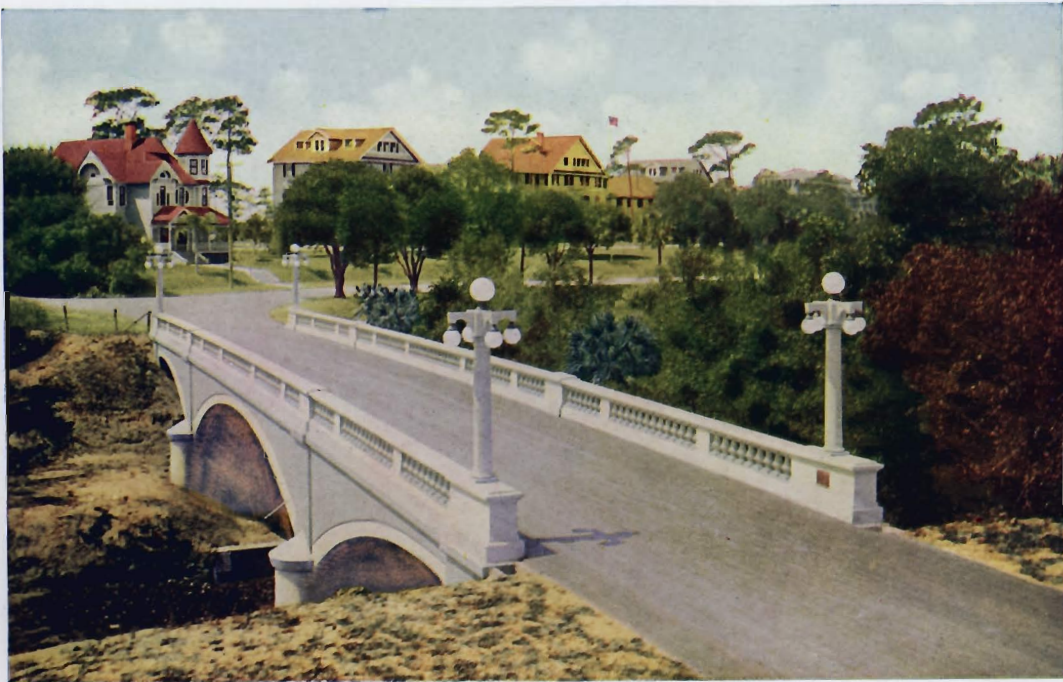
BELLEVUE BRIDGE, BELLEAIR, FLORIDA Three spans of 30 to 60 feet. Roadway 18 feet. Footings on sand. For M. F. Plant, New London, Connecticut, 1915. The end spans are half-arches, not cantilevers.
