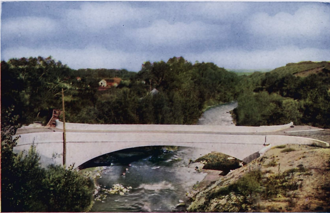
SEVENTEENTH STREET BRIDGE, BOULDER, COLORADO Span of waterway 70 feet. Roadway 24 feet. Footings in gravel with tie-plate. For the City of Boulder, Colorado, 1906.
