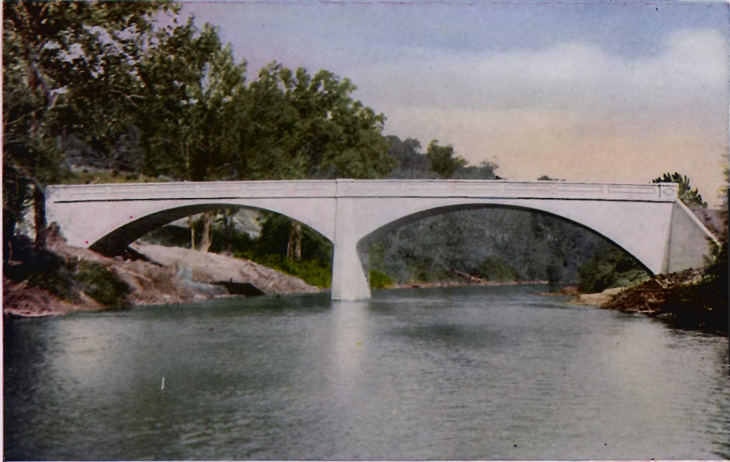
VONORE BRIDGE OVER TELLICO RIVER, VONORE, TENNESSEE Twin spans of 65 feet each. Roadway 16 feet. Footings on rock. For the Monroe County Road Commission. Madisonville, Tennessee, 1913. Illustrating thin pier, 4 feet at springing, 5 feet at base, for 75 ton load on one span.
