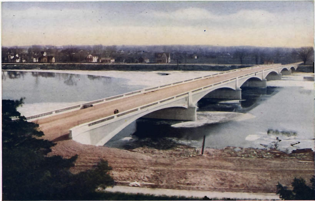
CICOTT STREET BRIDGE OVER WABASH RIVER, LOGANSPORT, INDIANA Six spans of 96 to 108 feet. Roadway 35 feet. Skew 20 degrees. Footings on rock. For the Board of Commissioners of Cass County, Logansport, Indiana, 1913. Replacing steel bridge destroyed in 1913 Easter Flood.
