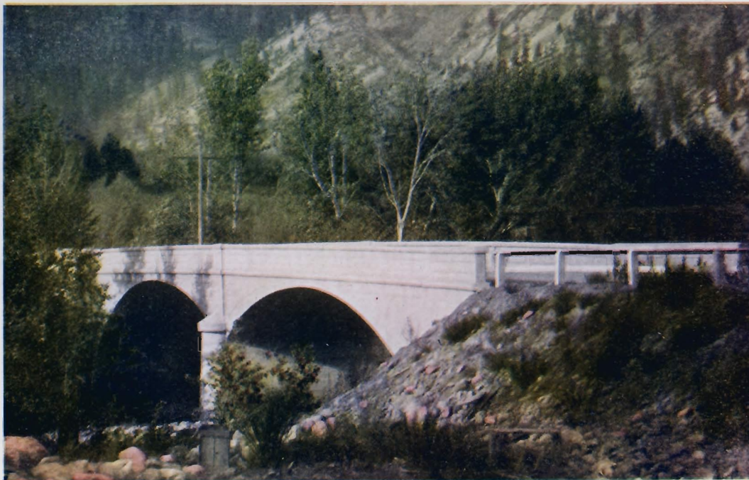
PESHASTIN CREEK BRIDGE, LEAVENWORTH, WASHINGTON Twin spans of 55 feet each. Roadway 20 feet. Footings on boulders. For the Board of Commissioners of Chelan County, Wenatchee, Washington, 1920.
