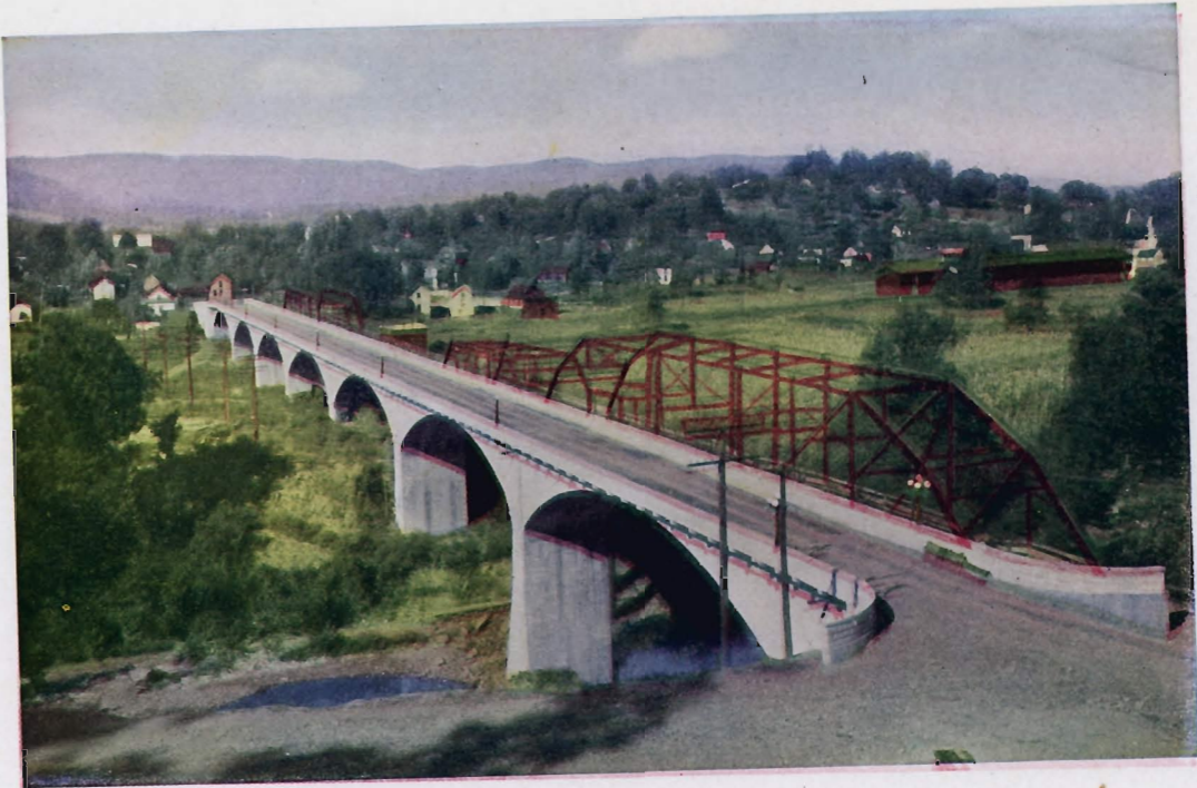
HARRIMAN BRIDGE OVER EMORY RIVER, HARRIMAN, TENNESSEE Seven spans of 85 to 120 feet. Roadway 24 feet. Footings on rock and on gravel. For the Bridge Committee of the City of Harriman, Tennessee, 1916.
