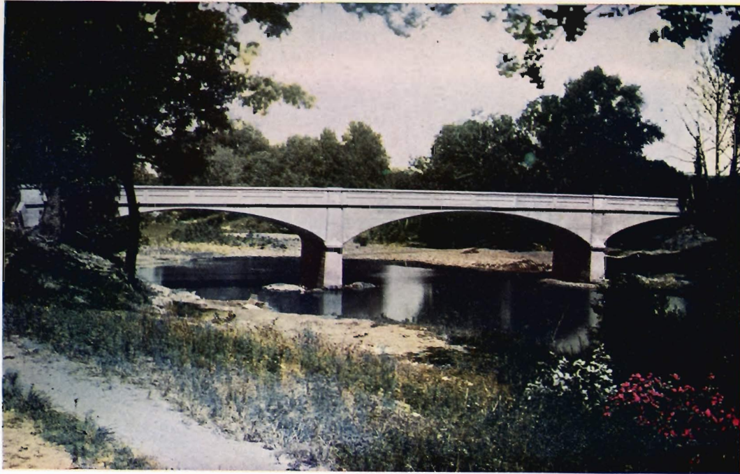
ELKINS BRIDGE OVER WHITE RIVER, WASHINGTON COUNTY, ARKANSAS Three spans of 62 to 68 feet. Roadway 16 feet. Footings on rock. For the Board of Commissioners of Washington County, Fayetteville, Arkansas.
