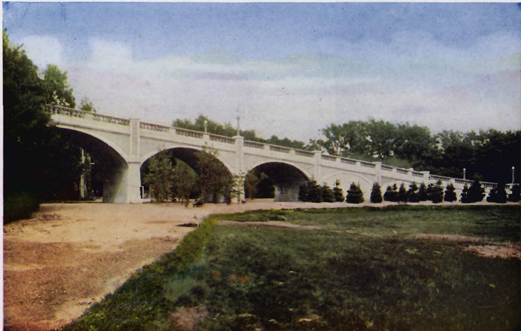
NORTON POINT BRIDGE, MANCHESTER-BY-THE-SEA, MASSACHUSETTS Six spans of 25 to 48 feet. Roadway 20 feet. Footings on clay. For William A. Tucker, New York City, 1912.
