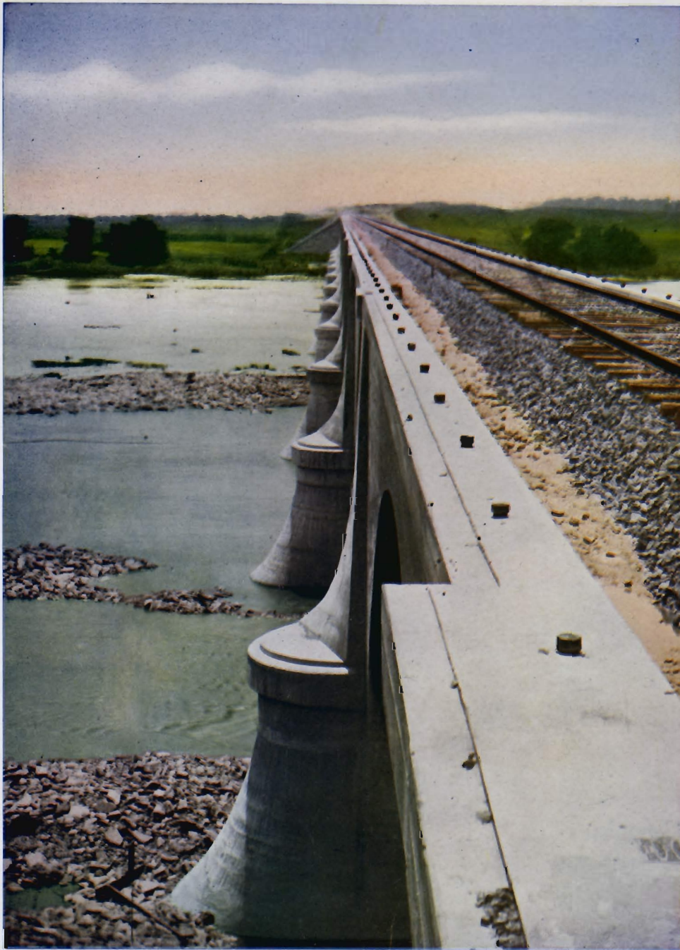
MAUMEE RIVER BRIDGE, WATERVILLE, OHIO. Twelve spans of 75 to 90 feet. Roadway 16 feet. Footings on rock. For the Ohio Electric Railway Company, Cincinnati, Ohio, 1907. Two additional views on page 8.
