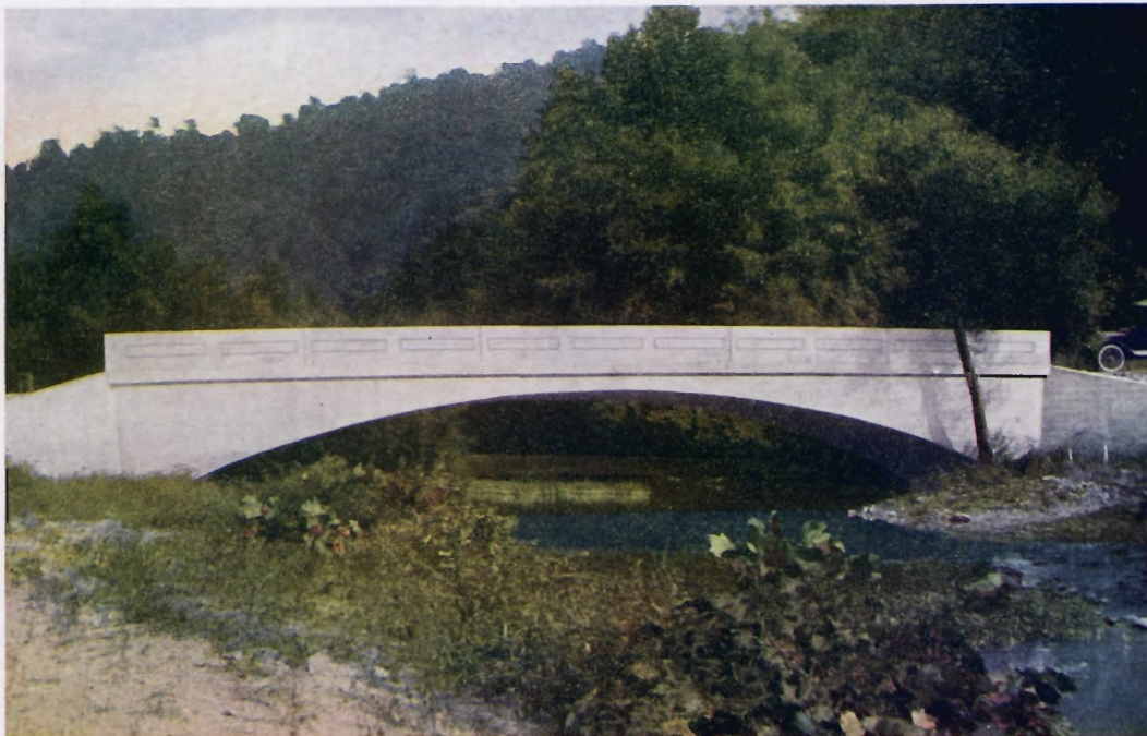
MEYERS BRIDGE, WETZEL COUNTY, WEST VIRGINIA Span of waterway 75 feet. Roadway 16 feet. Footings on gravel. For the County Court of Wetzel County, New Martinsville, West Virginia, 1919.
