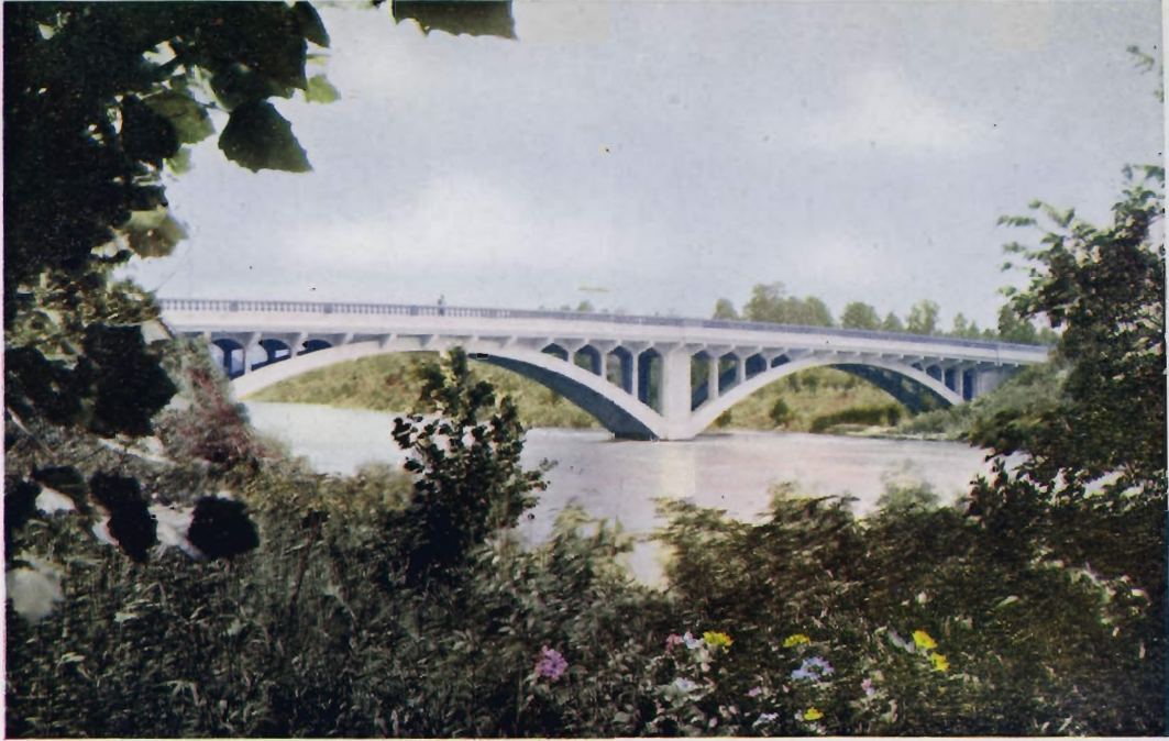
MT. AETNA BRIDGE OVER WABASH RIVER, HUNTINGTON, INDIANA Twin spans of 100 feet each. Roadway 24 feet. Footings on rock. For the Board of Commissioners of Huntington County, Huntington, Indiana, 1918. Open spandrel arches.
