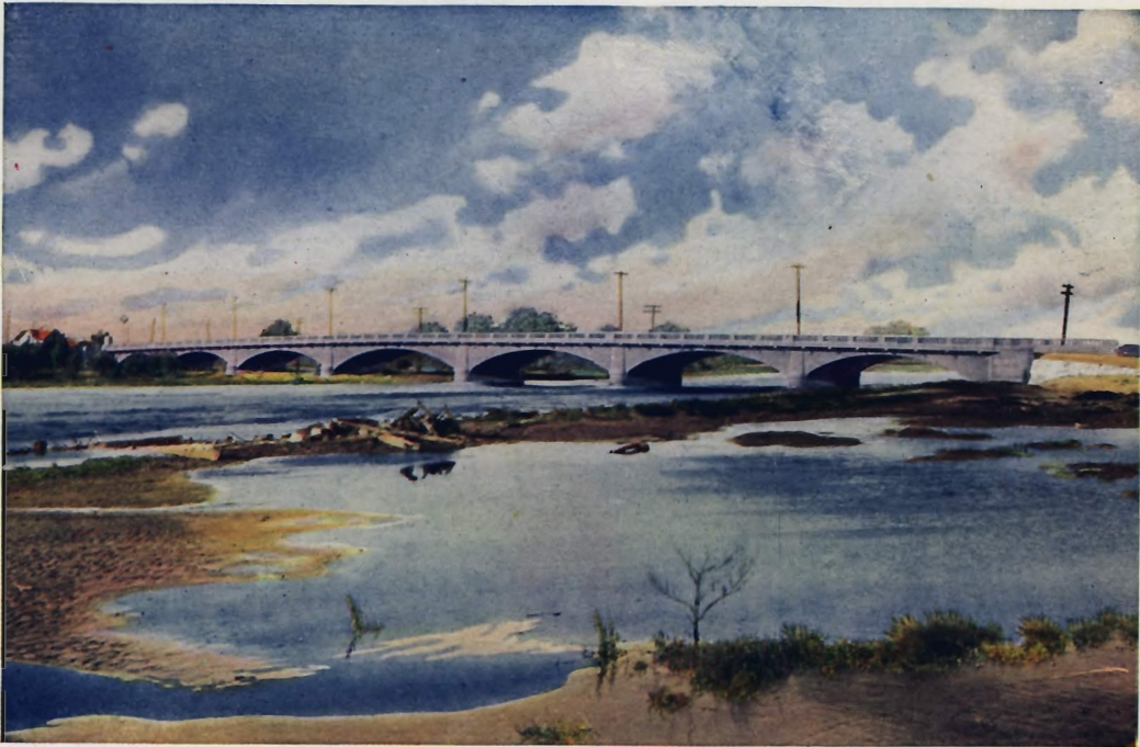
LA JUNTA BRIDGE OVER ARKANSAS RIVER, LA JUNTA, COLORADO Seven spans of 60 to 90 feet. Roadway 24 feet. Footings on shale. For the Board of Commissioners of Otero County, La Junta, Colorado, 1914. This bridge was submerged to the hand rails in the 1921 Flood, without damage.
