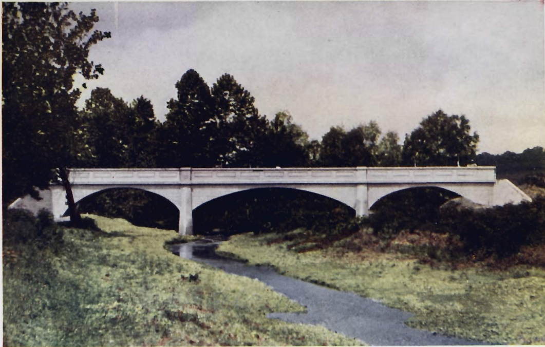
CLEAR CREEK BRIDGE, WASHINGTON COUNTY, ARKANSAS
