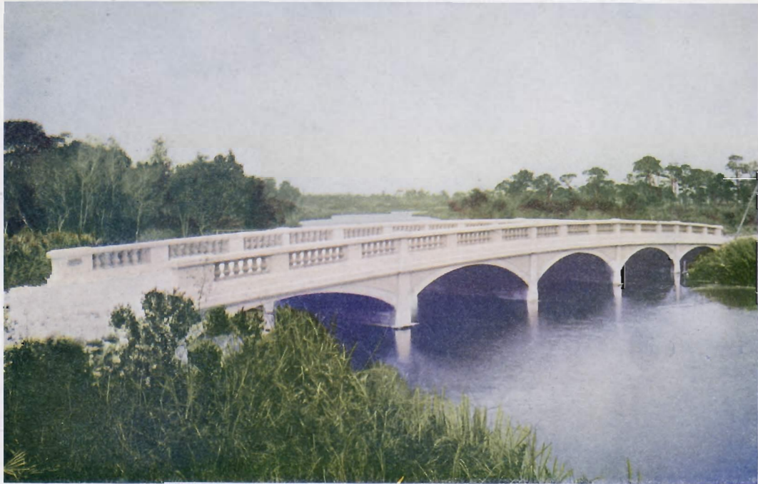
BIG SNAKE CREEK BRIDGE, DADE COUNTY, FLORIDA Five spans of 26 feet each. Roadway 16 feet. Footings on piling in sand. For the Board of Commissioners of Dade County, Miami, Florida, 1917.
