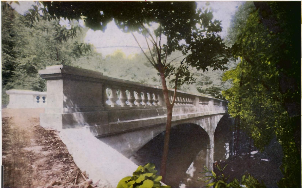
BUCKINGHAM BRIDGE, LAKE FOREST, ILLINOIS Three spans of 45 feet each. Roadway 36 feet. Footings on clay. For the Town of Lake Forest, Illinois, 1912. Illustrating details of concrete baluster hand rail.
