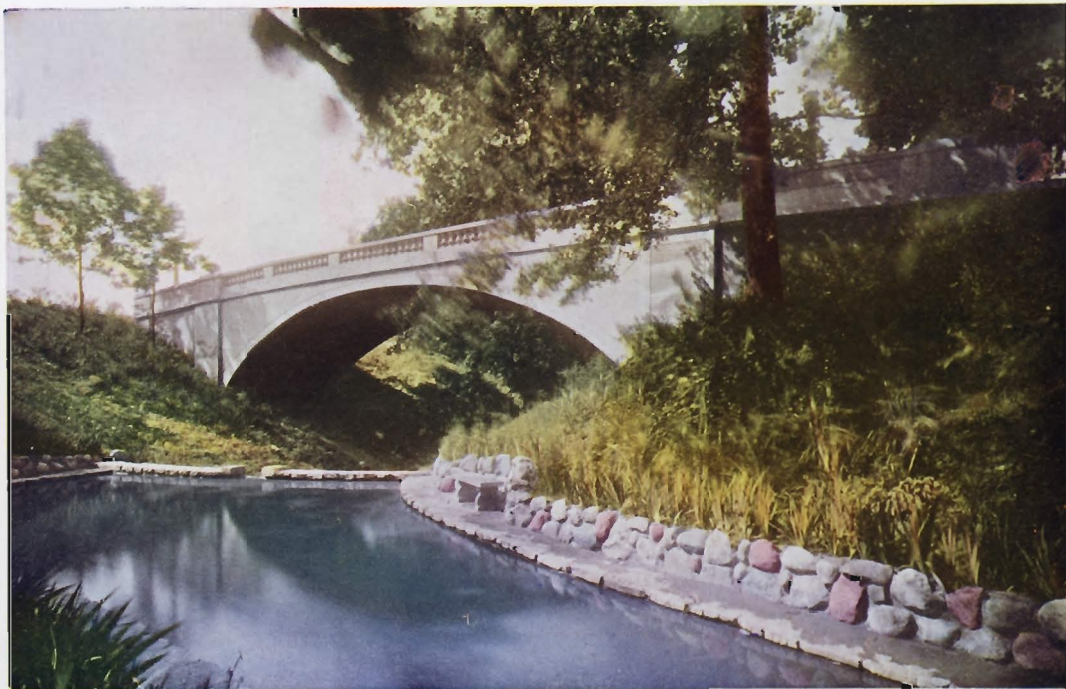
DOUBLE-DRUM ARCH ON J. I. HOLCOMB ESTATE, INDIANAPOLIS, INDIANA Span of opening 60 feet. Roadway 18 feet. Footings on loam. For J. I. Holcomb, Indianapolis, Indiana, 1919. Earth-filled arch having two four-inch rings with tamped earth between.
