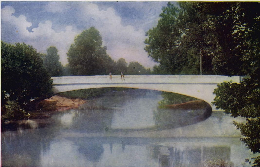
YORKTOWN BRIDGE OVER BUCK CREEK, YORKTOWN, INDIANA Span of waterway 95 feet. Roadway 16 feet. Footings in gravel with tie-plate. For the Board of Commissioners of Delaware County, Muncie, Indiana, 1904.
