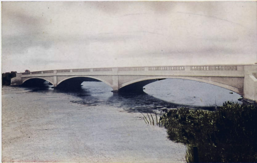
TIDEWATER BRIDGE OVER BIG SNAKE CREEK, DADE COUNTY, FLORIDA Three spans of 60 feet each. Roadway 18 feet. Footings on piling in sand. For the Board of Commissioners of Dade County, Miami, Florida, 1917.
