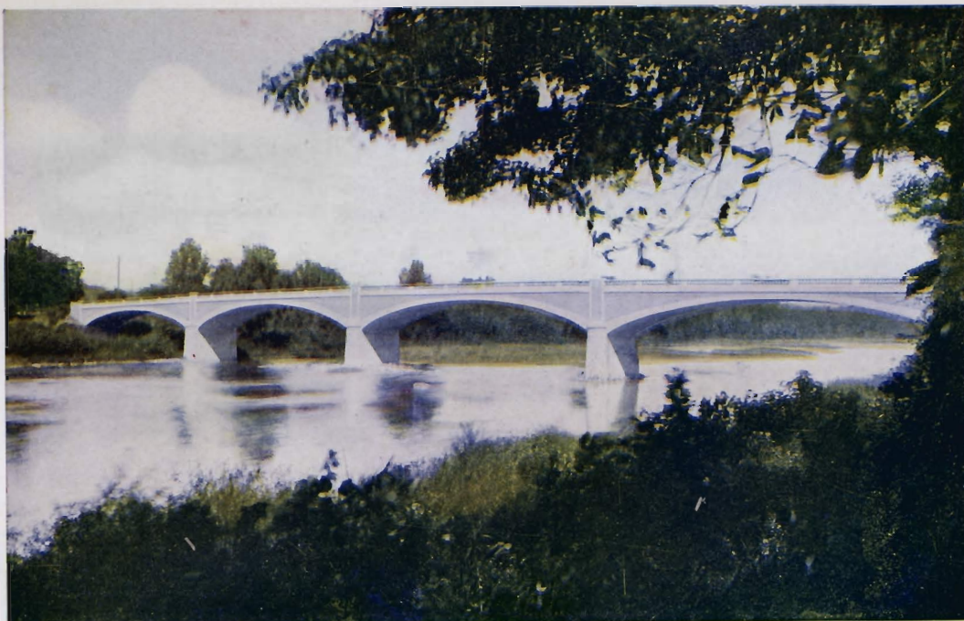
ZIMMERMAN BRIDGE OVER WABASH RIVER, COUNTRY CLUB, LOGANSPORT, INDIANA Four spans of 110 feet each. Roadway 20 feet. Footings on rock. For the Board of Commissioners of Cass County, Logansport, Indiana, 1917.
