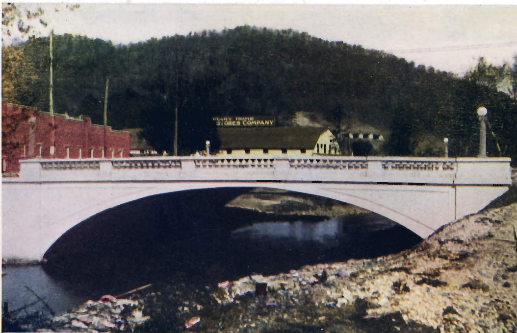
CENTRAL AVENUE BRIDGE OVER INDIAN CREEK, LAFOLLETTE, TENNESSEE Span of waterway 64 feet. Roadway 58 feet. Footings on rock. For the Board of City Commissioners, LaFollette, Tennessee, 1921.
