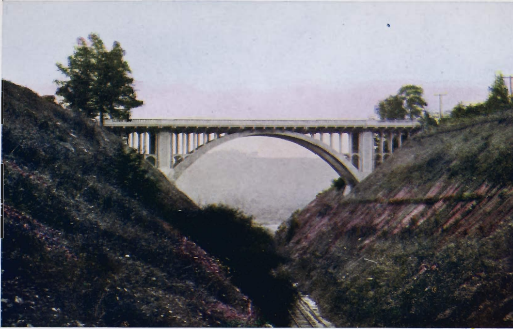
COLWELL CUT BRIDGE OVER PITTSBURG & SHAWMUT R. R., COLWELL, PENNSYLVANIA Span of opening 128 feet. Roadway 24 feet. Footings on shale. For the Pittsburg & Shawmut Railroad Company, Kittanning, Pennsylvania, 1921.
