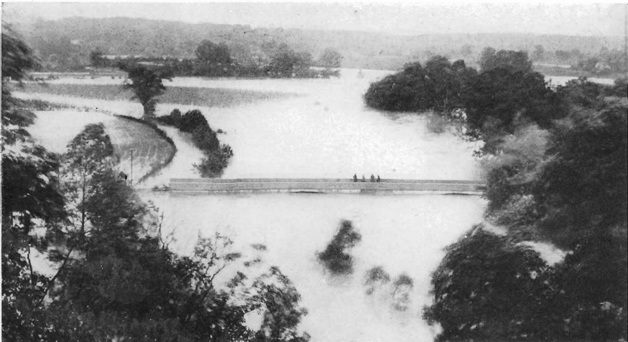
FREDERICKSBURG BRIDGE, SALEM, INDIANA Showing the same bridge at top of page in 1913 Easter Flood. No damming of river, no obstruction to debris. Debris is deflected by the water cushion at the haunches to the crowns of the arches. Water level at end of bridge at left shows that the bridge is discharging the entire flood.
