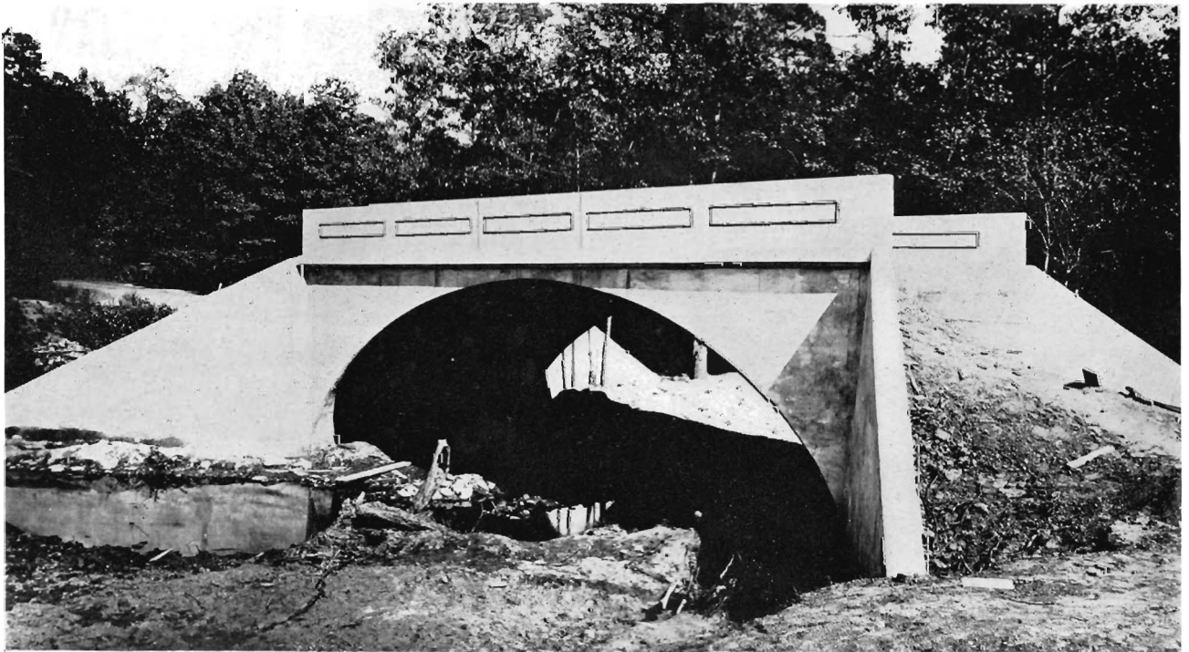
FOE-KILLER CREEK BRIDGE, MILTON COUNTY, GEORGIA Span of waterway 40 feet. Roadway 20 feet. Footings on rock. For the Commissioners of Milton County and the State Highway Department, Atlanta, Georgia, 1919. Federal Aid Project No. 22. This was the first Federal Aid Bridge built in Georgia.
