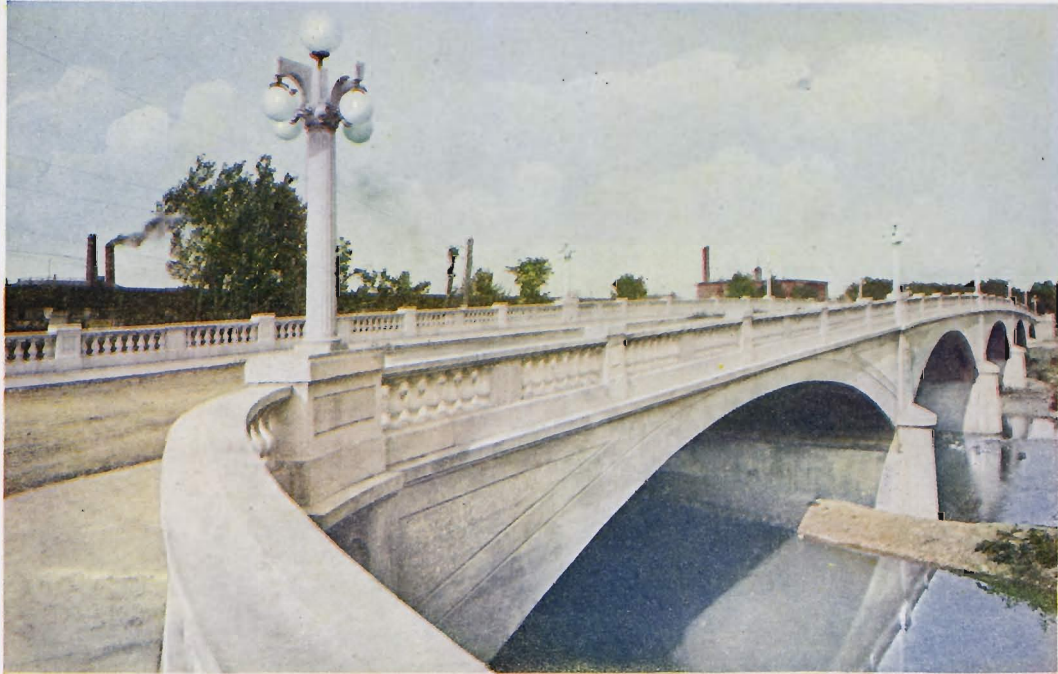
SHAWNEE BRIDGE ON UNION STREET, OVER GREAT MIAMI RIVER, PIQUA, OHIO Five spans of 94 to 110 feet. Roadway 50 feet. Footings on piling in gravel. For the Board of Commissioners of Miami County, Troy, Ohio, 1914.
