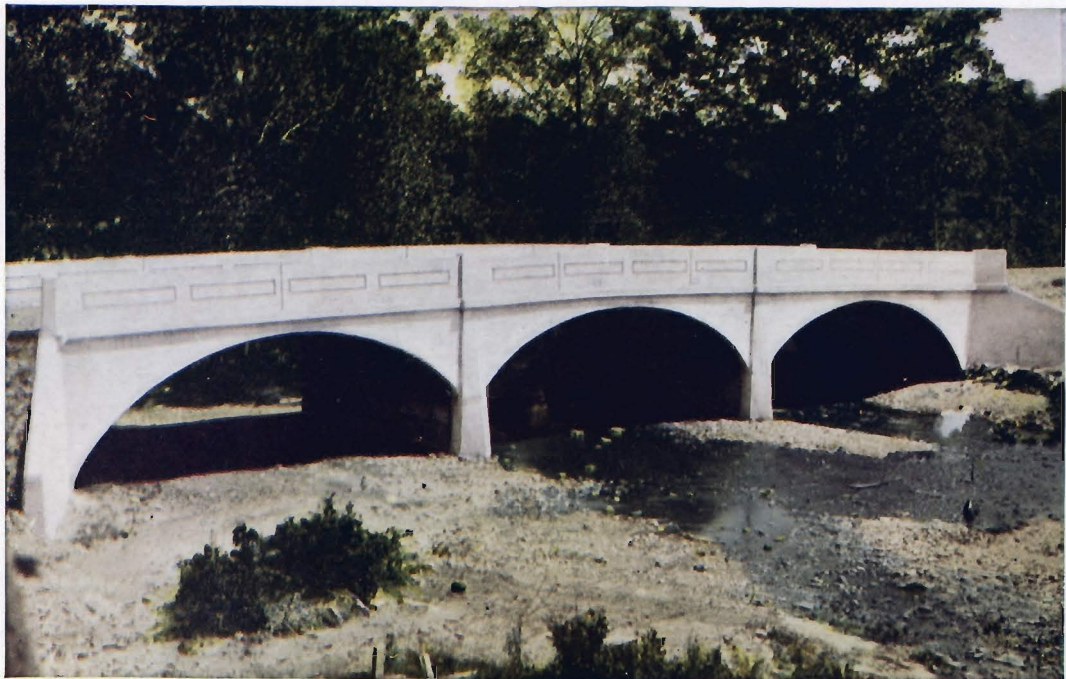
ROCK CREEK BRIDGE, MURRAY COUNTY, GEORGIA Three spans of 30 feet each. Roadway 18 feet. Footings on rock. For the Board of Commissioners of Murray County, and the State Highway Department, Atlanta, Georgia, 1921. Federal Aid Project No. 190.
