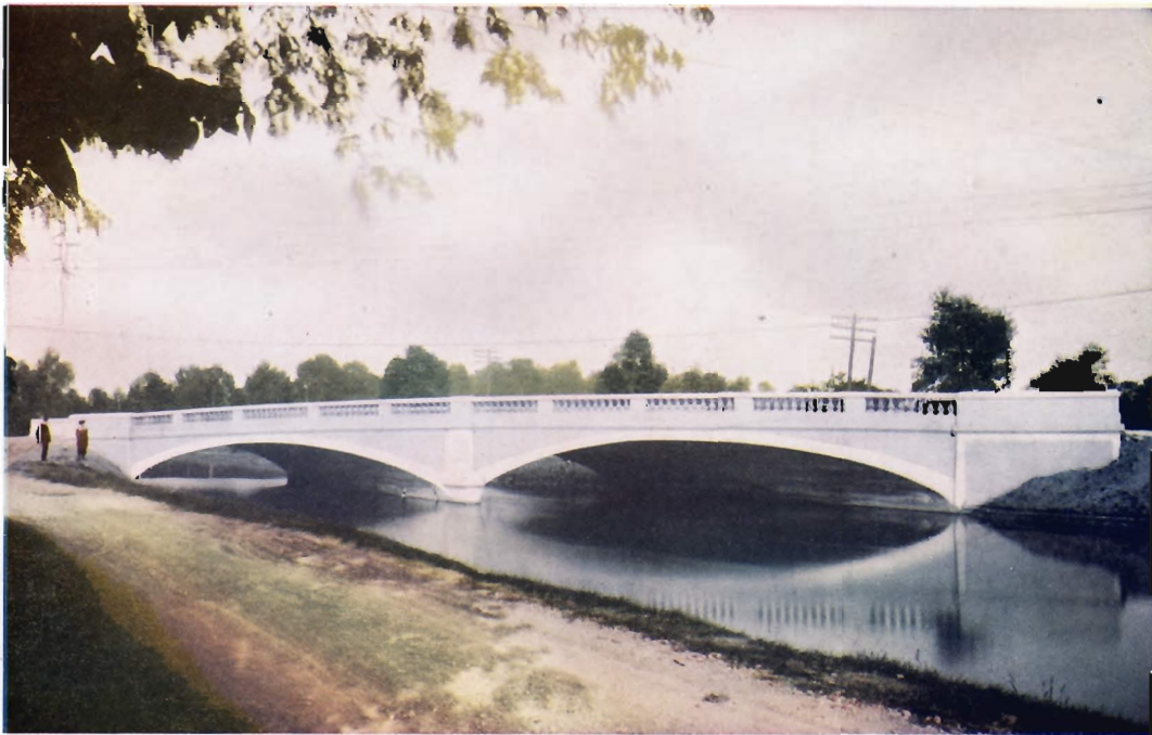
ILLINOIS STREET BRIDGE OVER WATER SUPPLY CANAL, INDIANAPOLIS, INDIANA Twin spans of 52\frac{1}{2} feet each. Roadway 24 feet. Skew 60 degrees. Footings on clay. For the Board of Commissioners of Marion County, Indianapolis, Indiana, 1920. Angle of crossing 30 degrees. Built with taper abutments by Royse formula.
