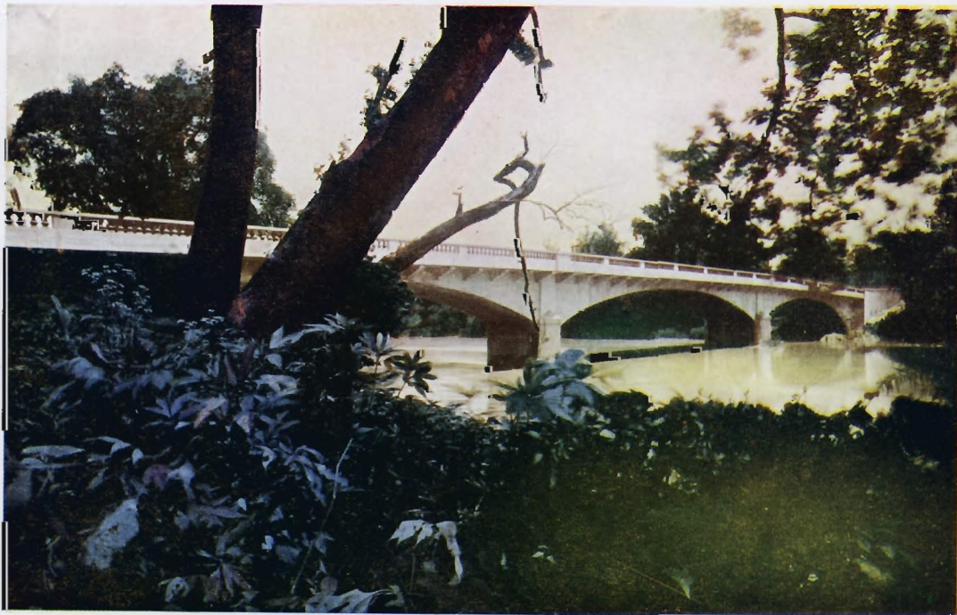
THIRD STREET BRIDGE OVER MISSISSINNEWA RIVER, MARION, INDIANA Three spans of 102 to 108 feet. Roadway 30 feet. Footings on hard-pan. For the Board of Commissioners of Grant County, Marion, Indiana, 1917.
