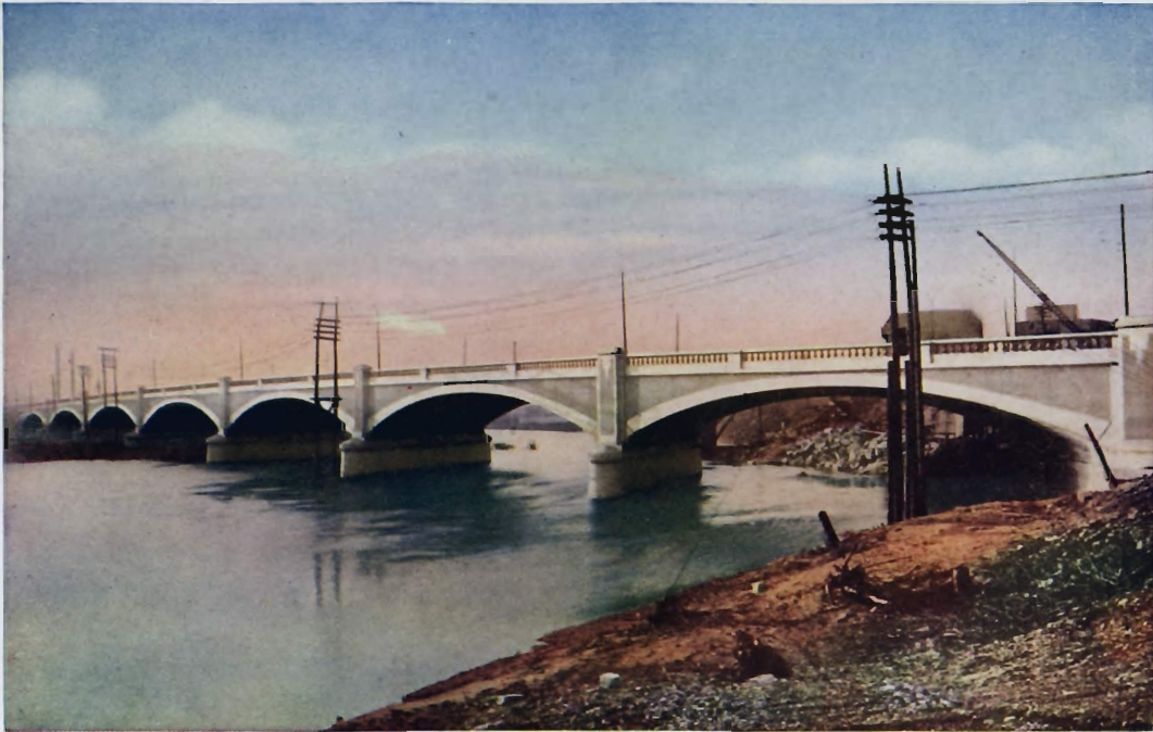
WEST WASHINGTON STREET BRIDGE OVER WHITE RIVER, INDIANAPOLIS, INDIANA Seven spans of 106 to 120 feet. Roadway 77 feet. Skew 30 degrees. Footings on piling in gravel. For the Board of Commissioners of Marion County, Indianapolis, Indiana, 1914-16. Earth-filled arches replacing steel bridge destroyed by the 1913 Easter Flood.
