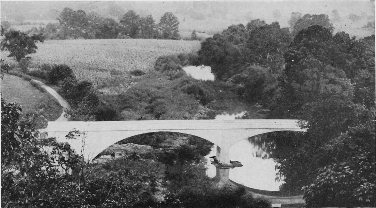
FREDERICKSBURG BRIDGE, SALEM, INDIANA Twin spans of 80 feet each. Roadway 16 feet. Footings on clay. For the Board of Commissioners of Washington County, Salem, Indiana, 1910. The view below shows the same bridge in 1913 Easter Flood.
