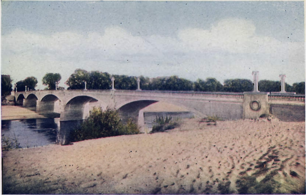
AMERICAN RIVER BRIDGE, SACRAMENTO, CALIFORNIA Five spans of 112 to 125 feet. Roadway 21 feet. Footings on piling in sand. For the Board of Supervisors of Sacramento County, Sacramento, California, 1915.
