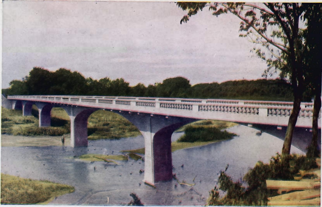
LITTLE BLUE RIVER BRIDGE, HANOVER, KANSAS Five spans of 65 to 70 feet. Roadway 18 feet. Footings on rock. For the Board of Commissioners of Washington County, Washington, Kansas, 1916. Cantilever slab at crowns, brackets at piers.
