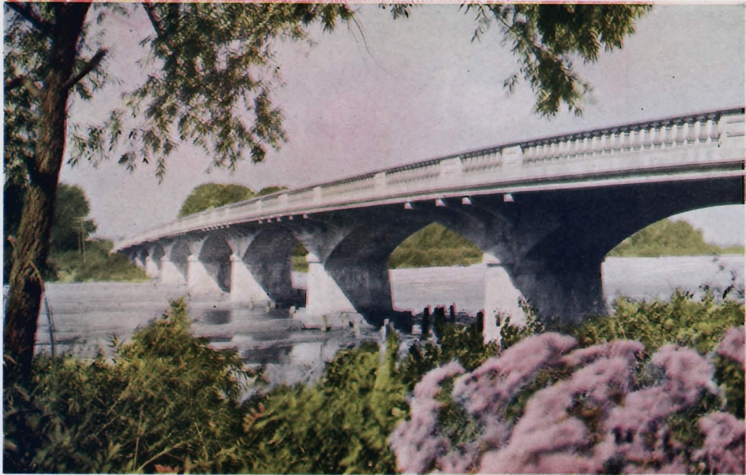
CHESTNUT STREET BRIDGE OVER ARKANSAS RIVER, ARKANSAS CITY, KANSAS Nine spans of 47 to 59 feet. Roadway 18 feet. Footings on cylindrical caissons to rock. For the Board of Commissioners of Cowley County, Kansas, 1914. Cantilevered slab at crown, brackets at piers for roadway, no sidewalks.
