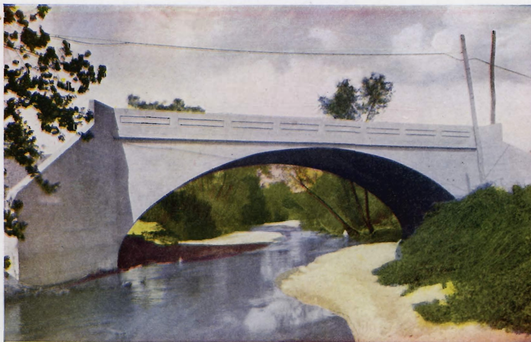
PROCTOR'S CREEK BRIDGE, FULTON COUNTY, GEORGIA Span of waterway 60 feet. Roadway 20 feet. Footings on rock. For the Board of Commissioners of Fulton County, Atlanta, Georgia, 1921
