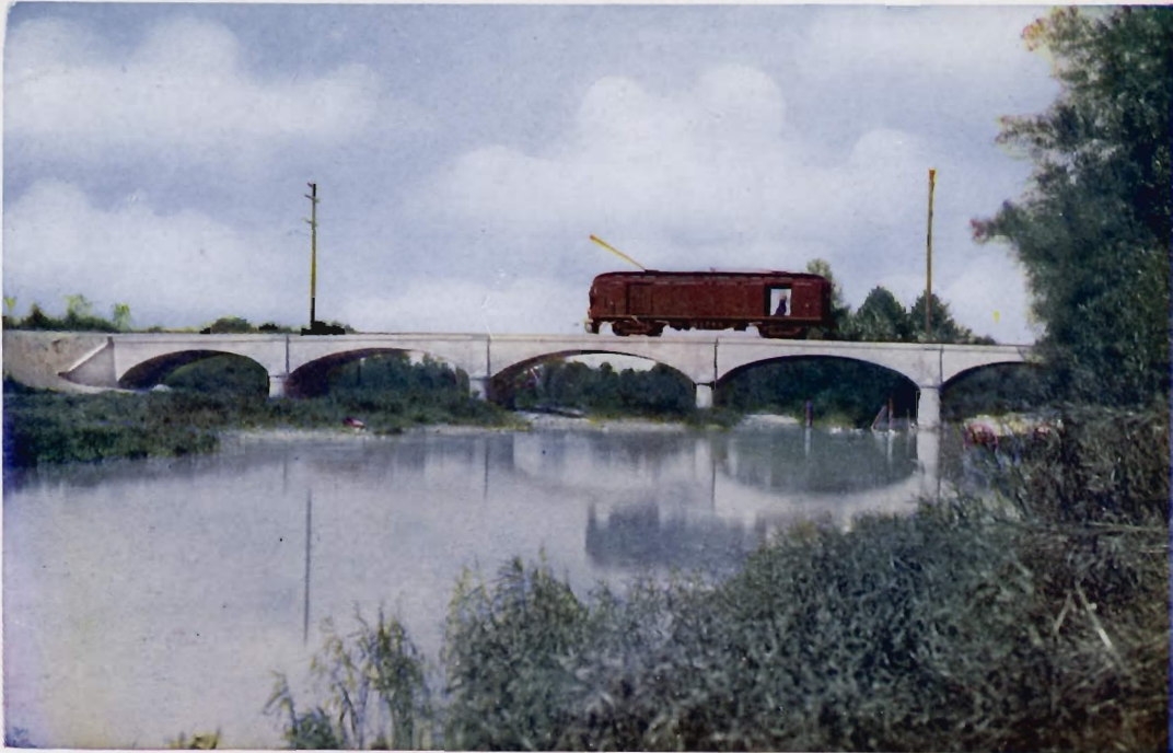
T. H., I. & E. RY. BRIDGE OVER WHITE LICK CREEK, PLAINFIELD, INDIANA Five spans of 35 to 42 feet. Roadway 16 feet. Footings on clay. For the Terre Haute, Indianapolis and Eastern Traction Company, Indianapolis, Indiana, 1906. Carries 60 ton cars; designed for 100 ton cars.
