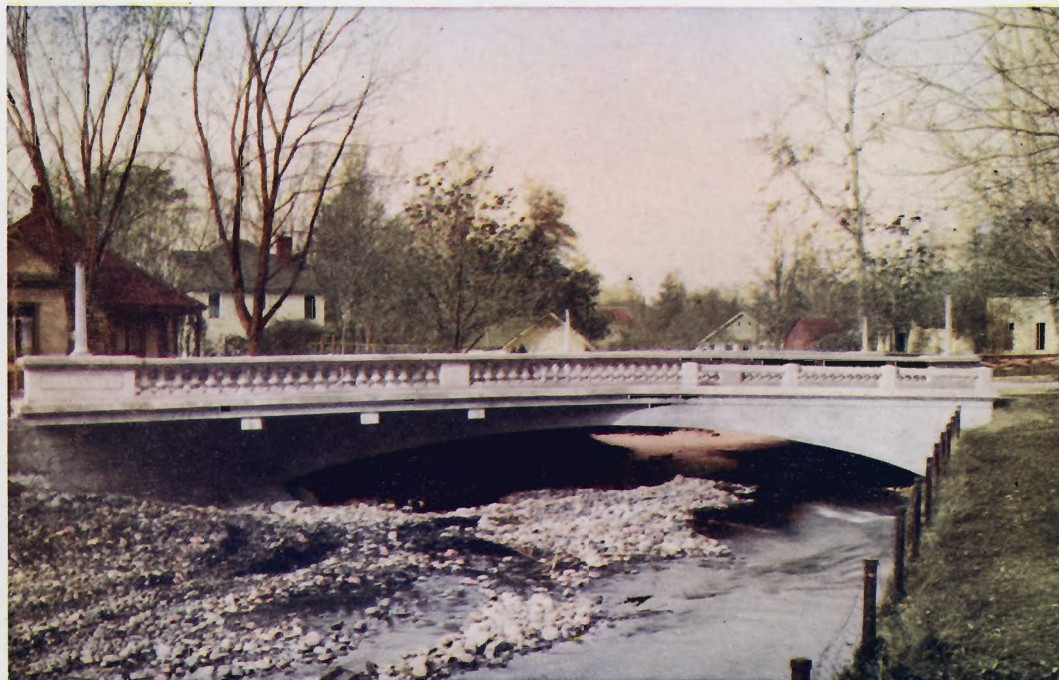
PARK STREET BRIDGE, WALLA WALLA, WASHINGTON Span of waterway 50 feet. Roadway 60 feet. Footings on cemented gravel. For the Commissioners of the City of Walla Walla, Washington, 1921. Arch square but roadway skewed on arch thirty degrees.
