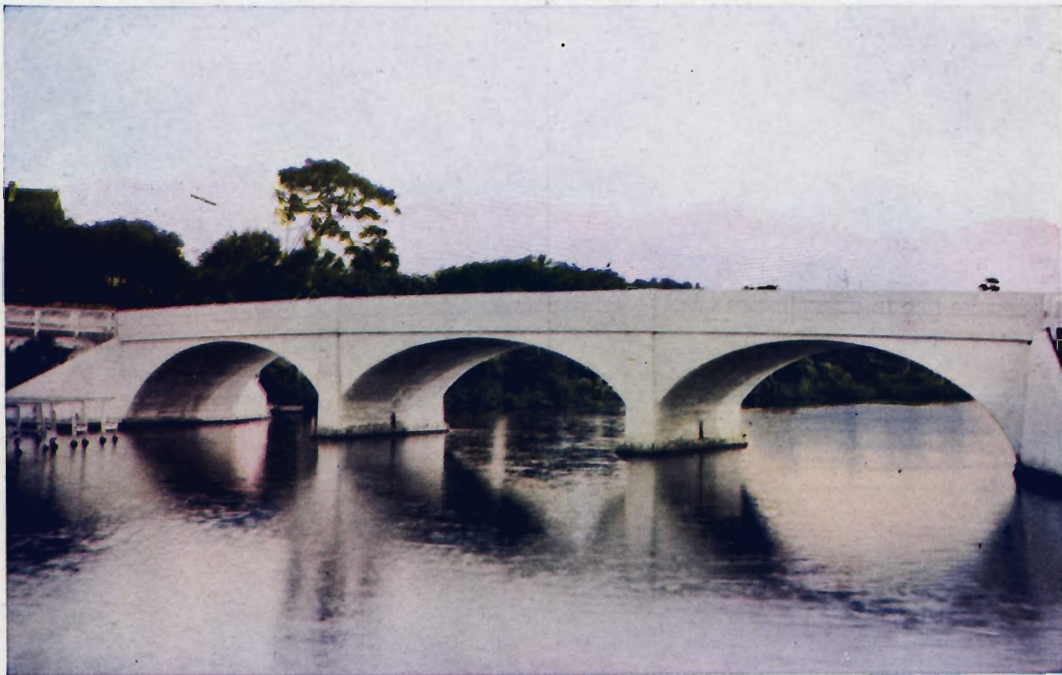
TILLMAN BRIDGE OVER TURKEY CREEK, BREVARD COUNTY, FLORIDA Three spans of 32 to 36 feet. Roadway 16 feet. Footings on piling in sand. For the Board of Commissioners of Brevard County, Titusville, Florida, 1919.
