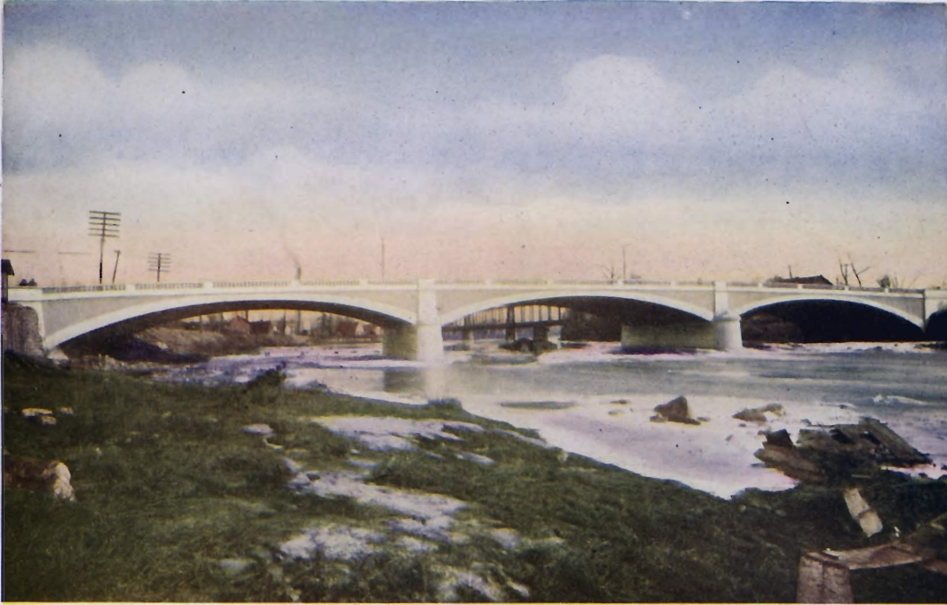
THIRD STREET BRIDGE OVER WABASH RIVER, LOGANSPORT, INDIANA Three spans of 96 to 101 feet. Roadway 49½ feet. Footings on rock. For the Board of Commissioners of Cass County, Logansport, Indiana, 1913. Carries 60 ton interurban cars. Replacing steel bridge destroyed in 1913 Easter Flood.
