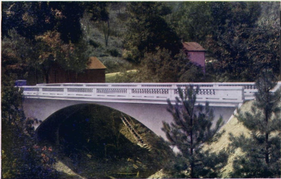
STERLING HEIGHTS BRIDGE OVER COAL RUN, FAIRMONT, WEST VIRGINIA Span of waterway 80 feet. Roadway 20 feet. Footings on rock. For the Sterling Heights Company, Fairmont, West Virginia, 1923. Spandrel braced arch.
