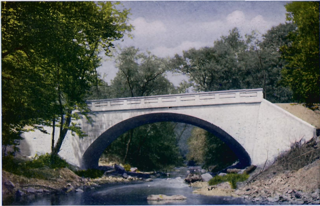
BLAIR BRIDGE OVER NORTHWEST BRANCH, MONTGOMERY COUNTY, MARYLAND Span of waterway 55 feet. Roadway 22 feet. Footings on gravel and clay. For the Maryland State Road Commission, Baltimore, Maryland, 1910.
