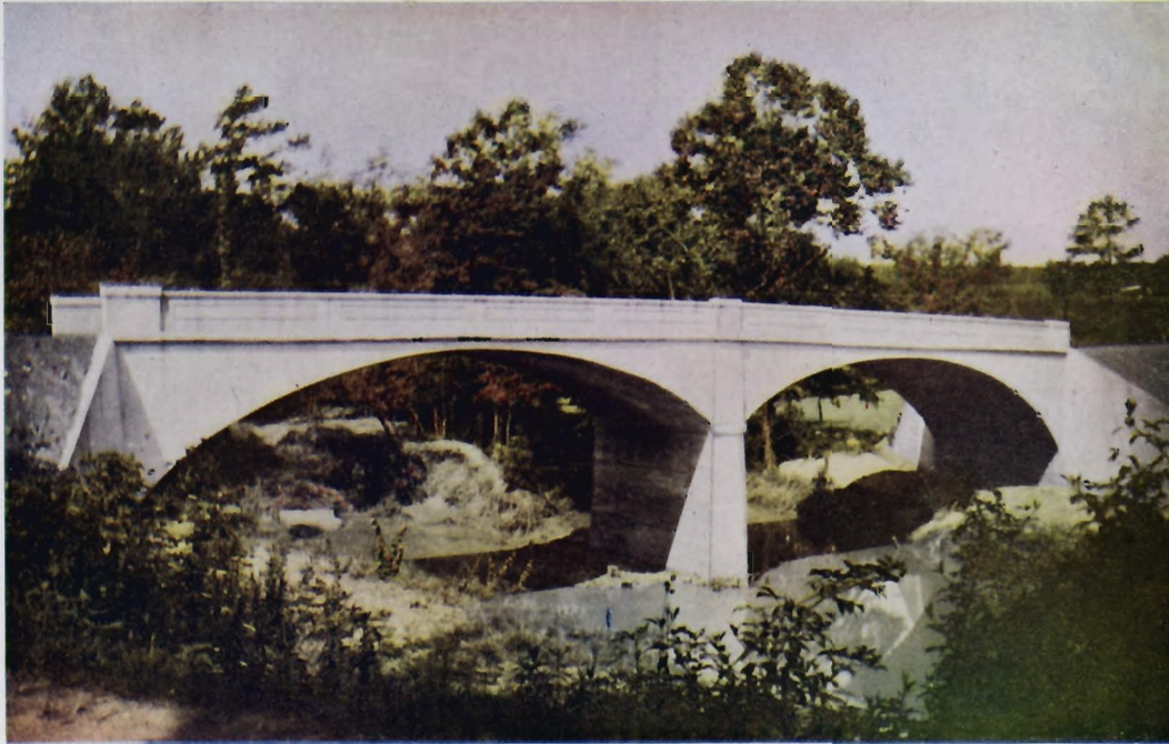
TWENTY-THREE MILE CREEK BRIDGE, ANDERSON COUNTY, SOUTH CAROLINA Twin spans of 55 feet each. Roadway 16 feet. Footings on rock. For the Anderson County Highway Commission, Anderson, South Carolina, 1920.
