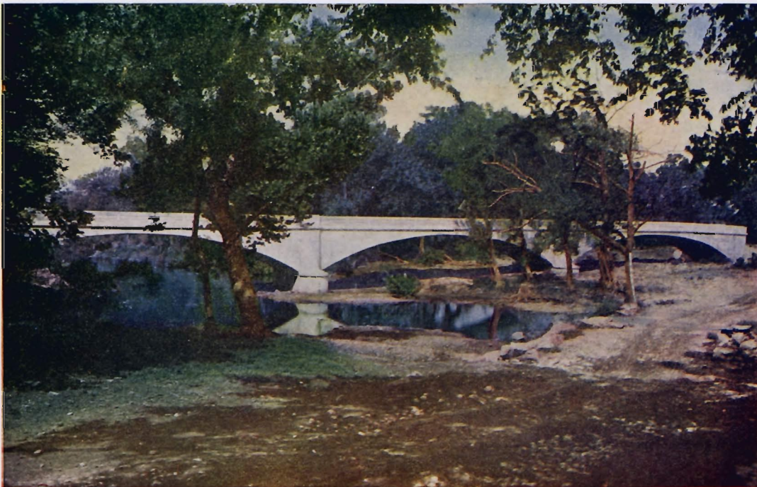
MINERS FORD BRIDGE, IOLA, KANSAS Three spans of 70 feet each. Roadway 16 feet. Footings in clay with tie-plate. For the Board of Commissioners of Allen County, Iola, Kansas, 1907.
