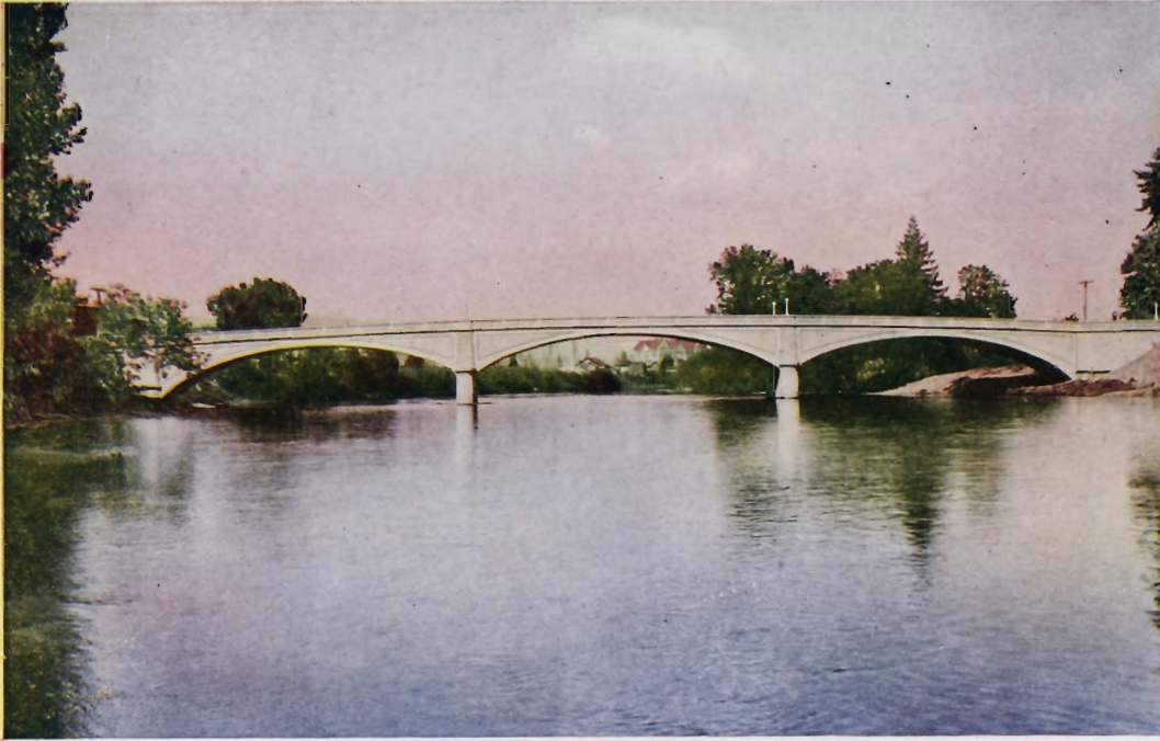
SNOQUALMIE RIVER BRIDGE, FALL CITY, WASHINGTON Three spans of 38 to 44 feet. Roadway 20 feet. Footings on clay. For the Board of Commissioners of King County, Seattle, Washington, 1916.
