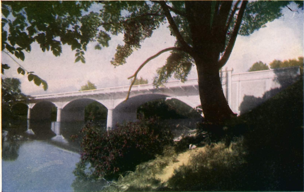
CENTENNIAL BRIDGE ON NORTHWESTERN AVENUE OVER WHITE RIVER, INDIANAPOLIS, INDIANA Five spans of 87 to 94 feet. Roadway 40 feet. Footings on piling in gravel. For the Board of Commissioners of Marion County, Indianapolis, Indiana, 1921. To commemorate the one hundredth anniversary of the founding of Indianapolis.
