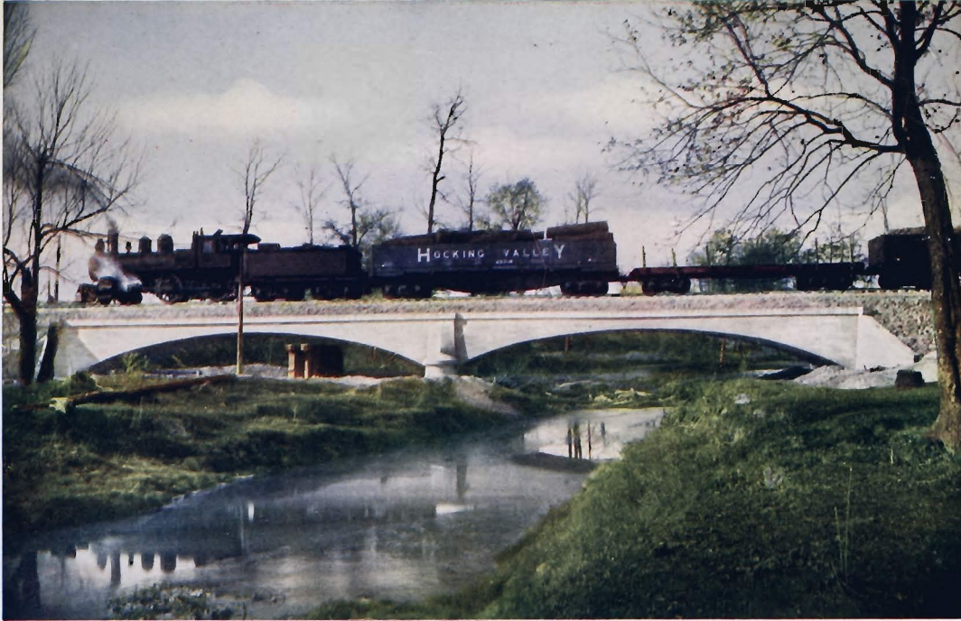
BRIDGE 816, C. & L. M. RY., OVER SUGAR CREEK, LIMA, OHIO Twin spans of 60 feet each. Roadway 22 feet. Footings on clay. For the Ohio Electric Railway Company, Cincinnati, Ohio, 1907. This bridge was built under the wooden truss that carried traffic during construction.
