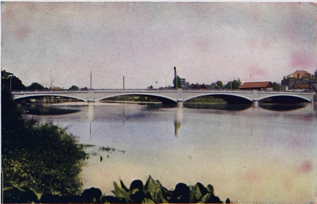
THIRD STREET BRIDGE OVER EEL RIVER, LOGANSPORT, INDIANA Four spans of 87 to 93 feet. Roadway 65 feet. Footings on rock. For the Board of Commissioners of Cass County, Logansport, Indiana, 1917.
