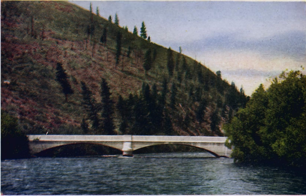
SHERWOOD BRIDGE OVER EAGLE RIVER, SHERWOOD, COLORADO Twin spans of 55 feet each. Roadway 16 feet. Footings on gravel. For the Board of Commissioners of Eagle County, Red Cliff, Colorado, 1913.
