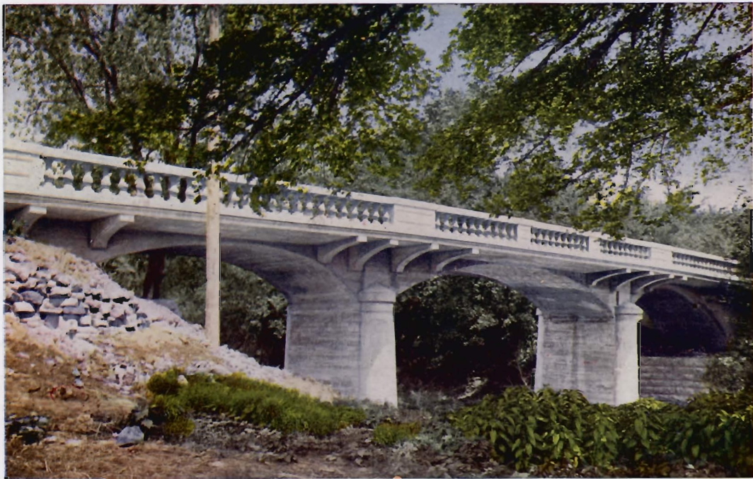
ISLAND PARK BRIDGE, WINFIELD, KANSAS Three spans of 35 to 45 feet. Roadway 24 feet. Footings on piling in sand. For the Board of Commissioners of Cowley County, Winfield, Kansas, 1912. Cantilever slab at crown, brackets at piers.
